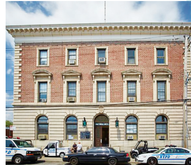
Historic building: NYPD 101st Precinct Police Station
