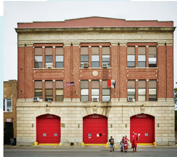
Historic building: Far Rockaway Firehouse, Engine Companies 264 & 328/Hook and Ladder 134
