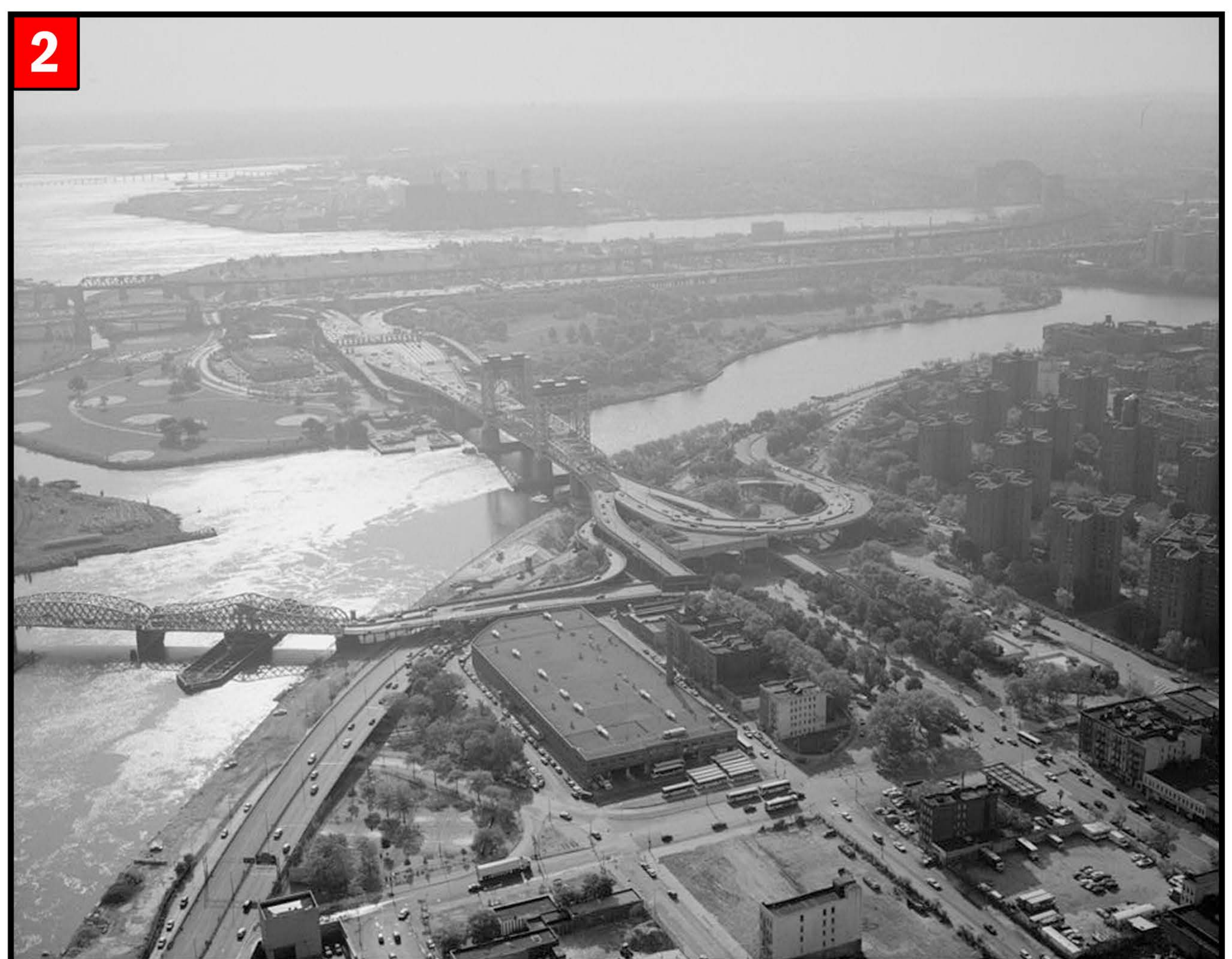
Aerial view of the bus depot looking East towards Randall's Island (Library of Congress).
