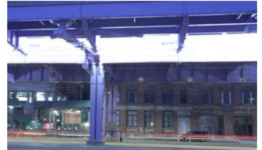
FDR Fascia Lighting
