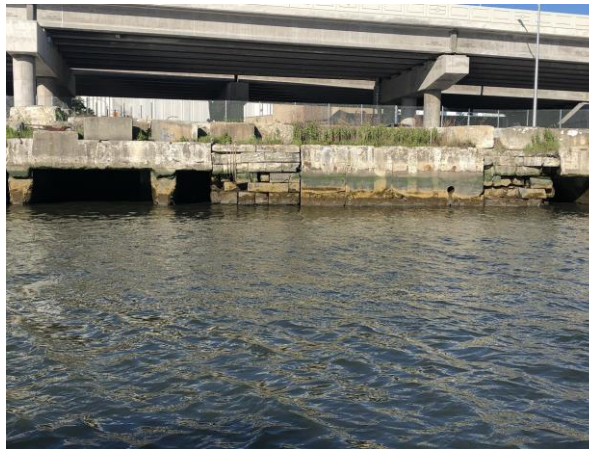
Bulkhead: The project features various types of bulkheads in different states of disrepair from 125 th all the way to Swindlers Cove
