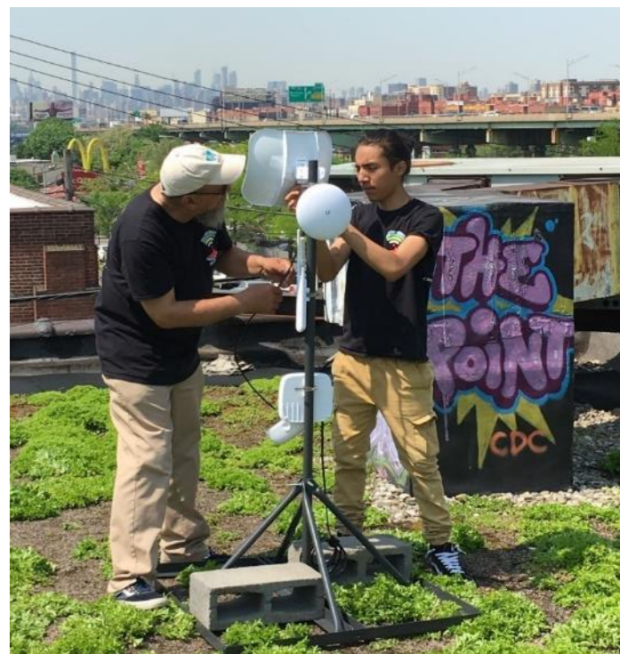
Hunts Point Digital Stewards configuring roof-top WiFi node
