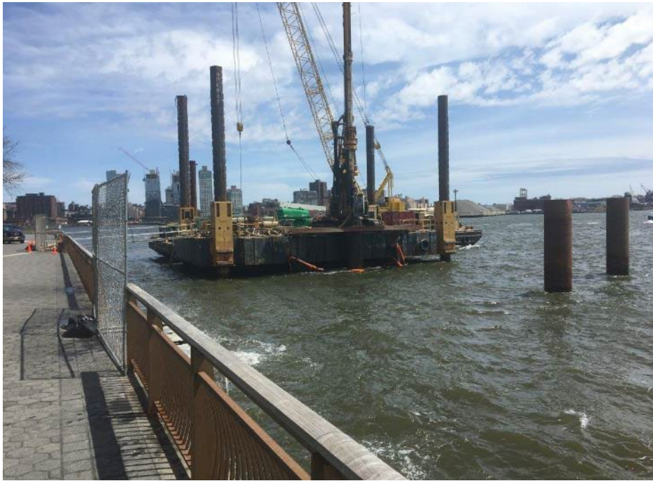
Barge mounted drill rig
