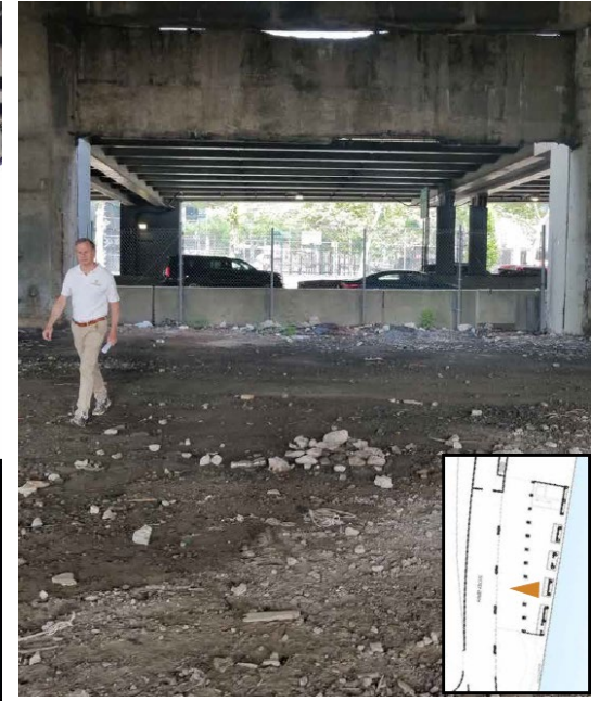
View looking West to FDR
