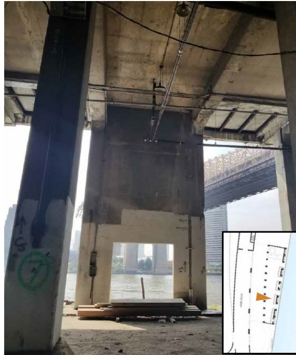
View looking East
