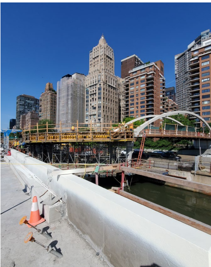
Formwork for waterside 54 th St. bridge ramp
