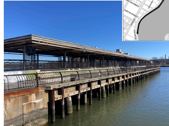
Existing Pier at 107 th St
