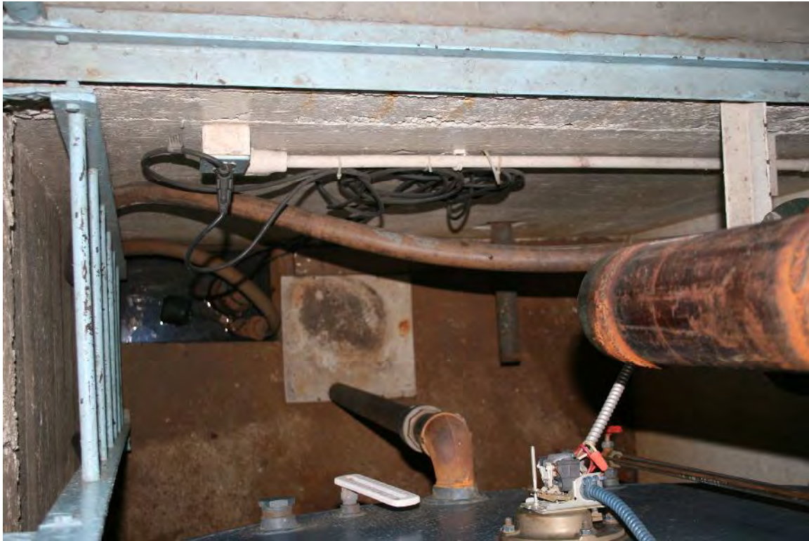
Photograph L: Boiler Room pit, in northwest corner of Boiler Room.
