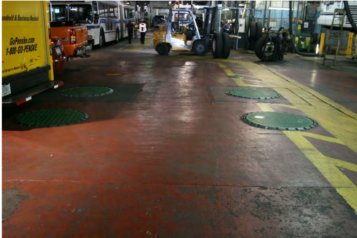
Photograph I: 8,000 gallon heat and oil tanks with green lids, excavated to ca.12 feet below grade, facing east.
