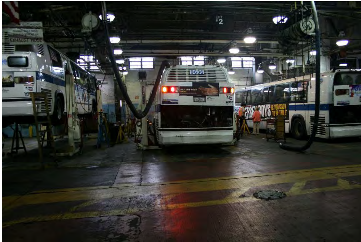
Photograph J: Former location of three in-ground lifts in Bus Lift Area facing south. Portions were excavated to ca.15 feet below grade.
