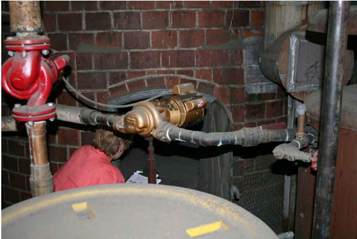
Photograph M: Base of chimney stack in Boiler Room, facing southeast.
