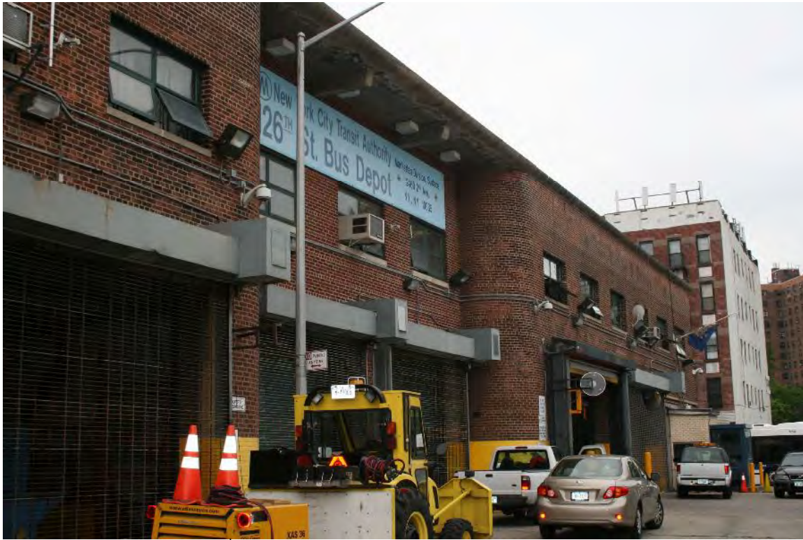
Photograph B: Façade of 126 th Street Bus Depot facing southeast from Second Avenue.
