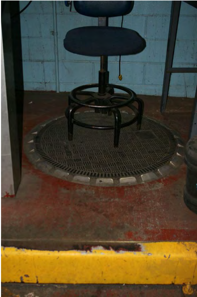
Photograph V: Manhole just outside Pump Room, facing northeast.
