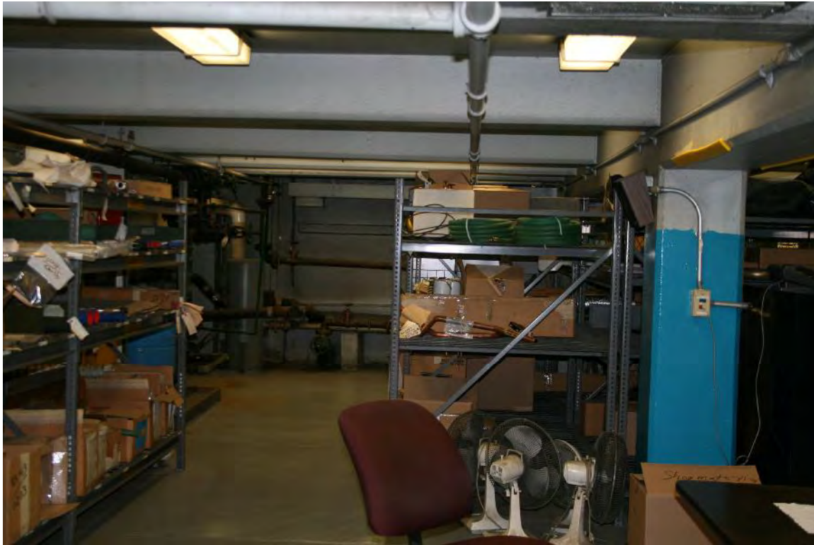
Photograph P: Below grade Store Room, facing south.
