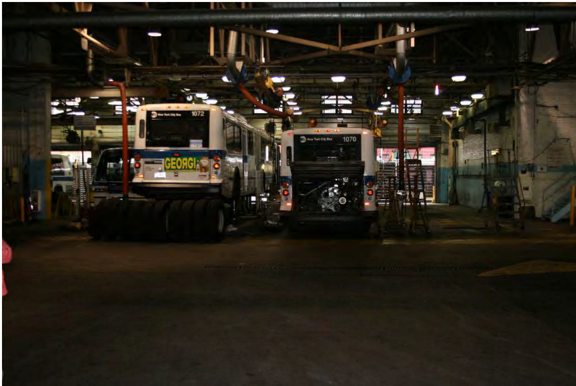
Photograph O: Three articulated three-pole lifts in West Maintenance Lift area, facing south. Entire lift area excavated to ca.20 feet below grade ca.1998.
