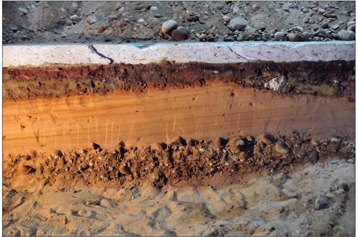
Saw-cut concrete foundation and clean, finely stratified glacial sands in the southern wall of Trench 1 7
