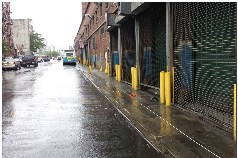
Facing west along southern face of bus depot. Trench 4 was excavated along sidewalk in the leftmost bay 4
