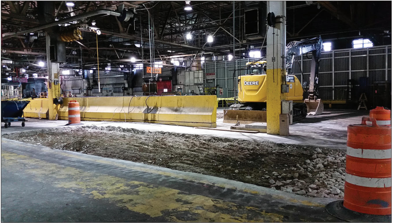
Looking north at Trench 1 after concrete removal and before excavation 1
