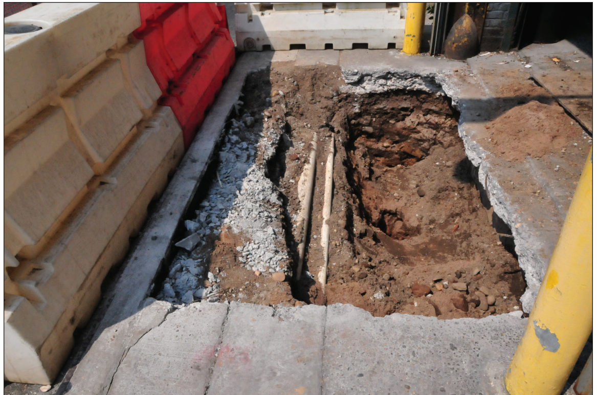
Facing west showing disturbed soils and existing infrastructure within Trench 4 18
