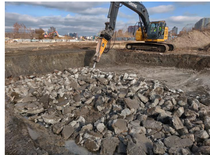
CONCRETE REMOVAL IN PETROLEUM IRM AREA
