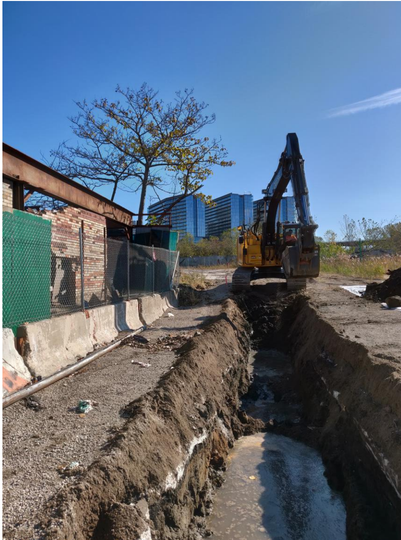
UST INVESTIGATION EXCAVATION AREA
