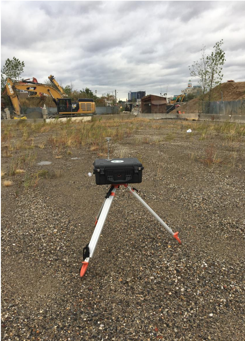
AIR MONITORING STATION
