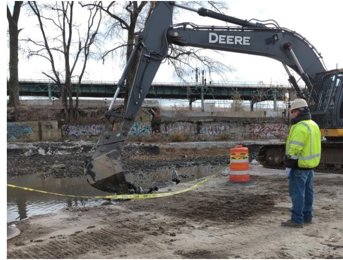
EXCAVATION WITHIN PETROLEUM IRM AREA
