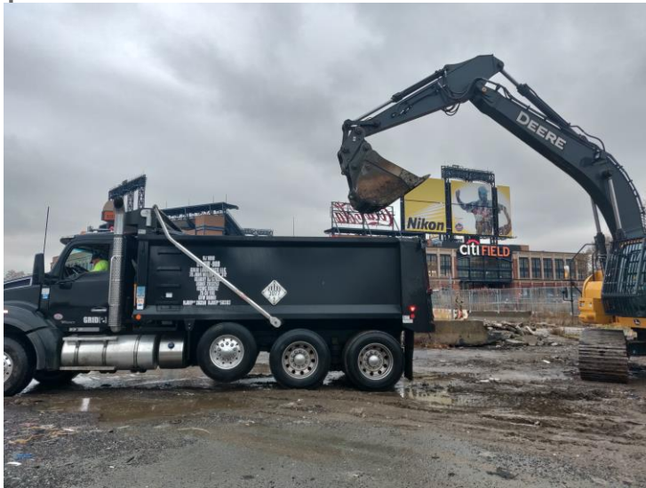
LOADING LEAD IMPACTED SOIL INTO TRUCK
