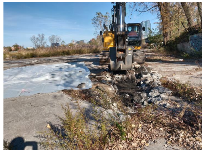
UST INVESTIGATION EXCAVATION AREA
