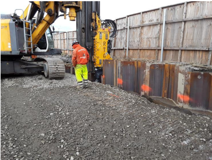
435 FEET OF GROUNDWATER CONTAINMENT WALL INSTALLED
