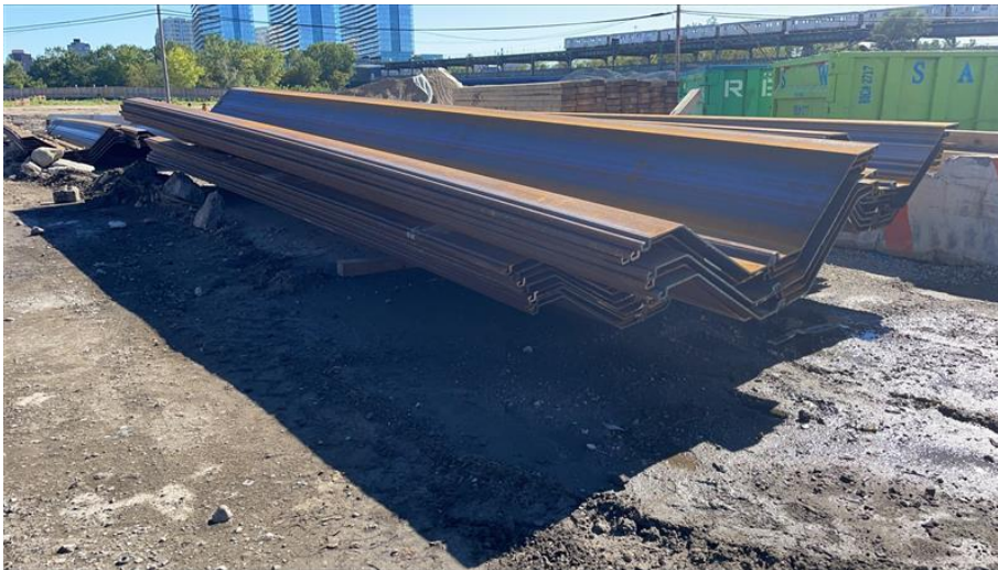
CONTAINMENT CUTOFF WALL SHEETING IMPORTED ONSITE
