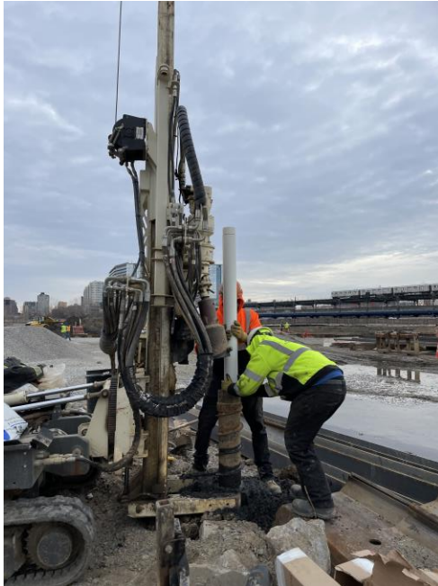
RECOVERY WELL INSTALLATION
