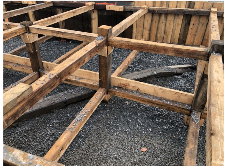
EXISTING UTILITY PROTECTION INSTALLED
