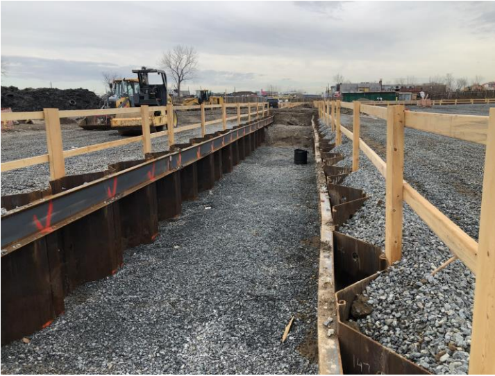
3,000 FEET OF SUPPORT-OF-EXCAVATION INSTALLED FOR FUTURE UTILITIES
