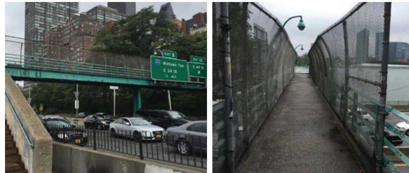
7. Pedestrian Bridge at 51st Street
