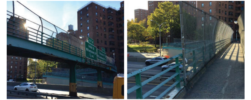
10. Pedestrian Bridge at 6th Street
