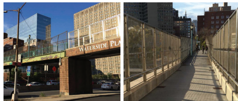
8. Pedestrian Bridge at 25th Street
