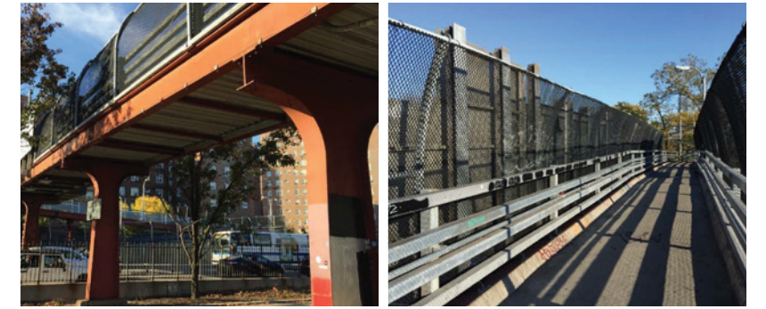
9. Pedestrian Bridge at 10th Street
