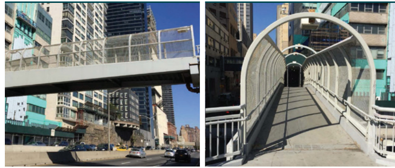
5. Pedestrian Bridge at 71st Street
