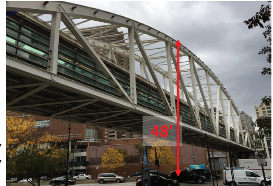
CHAMBERS STREET Span: ~230' Height: ~48'
