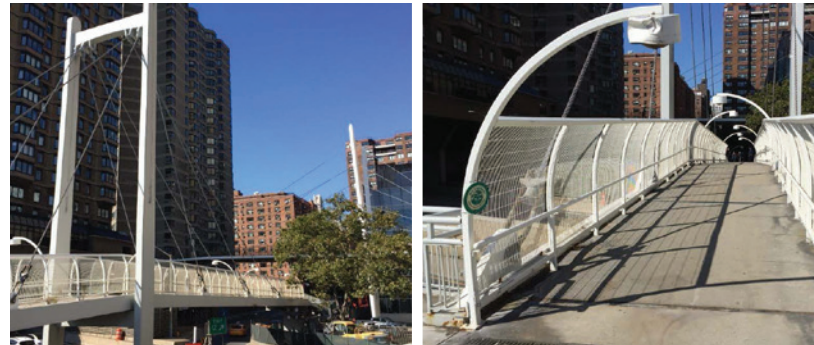
6. Pedestrian Bridge at 63rd Street
