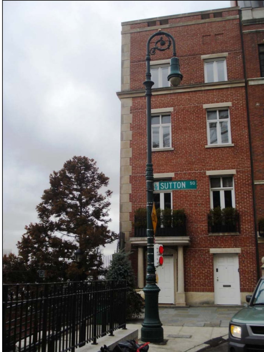
1 2 Photo 4 View looking south toward NYCLPC-designated Lamppost at the east end of East 58 th 3 Street. Note that original Twin F-type Lamppost was replaced in early 2000s with a replica 4 Bishop's Crook Lamppost (Number 6 on Figure 6-1). 5 6
