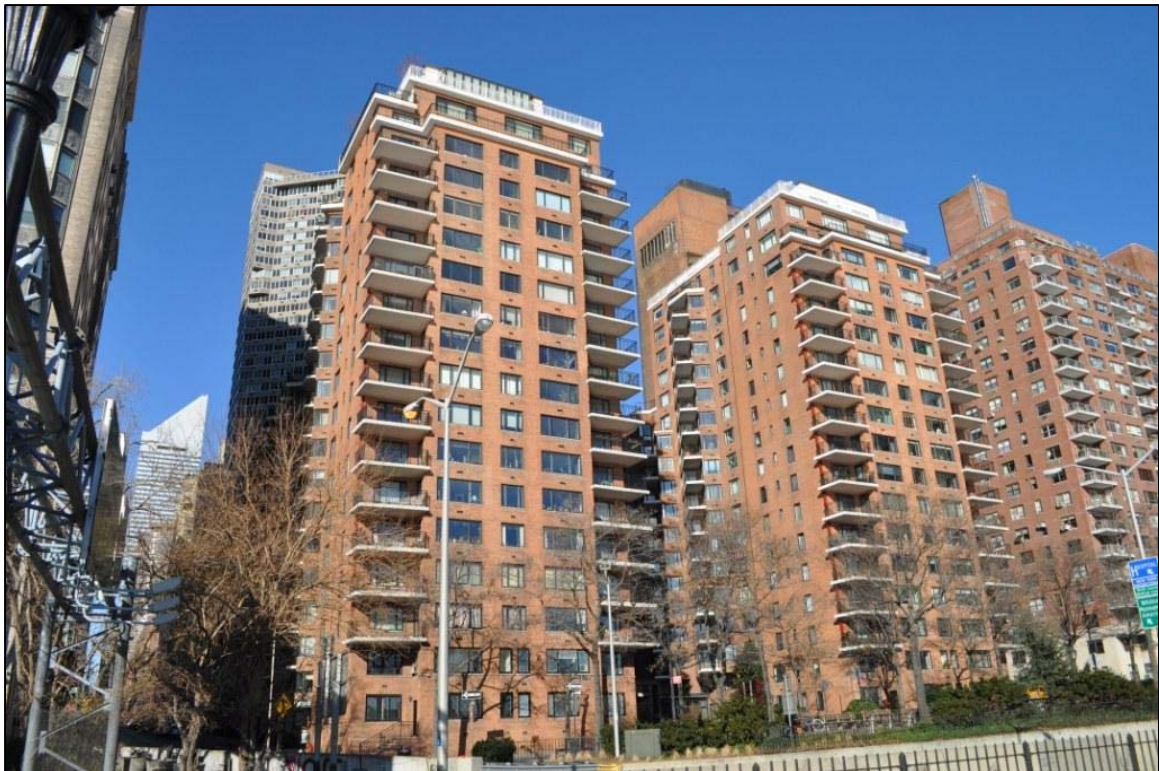
1 2 3 Photo 28 View looking west toward 60 Sutton Place South, a commonplace mid-century apartment building that lacks historical and architectural significance (Number 15 on Figure 6-1).
