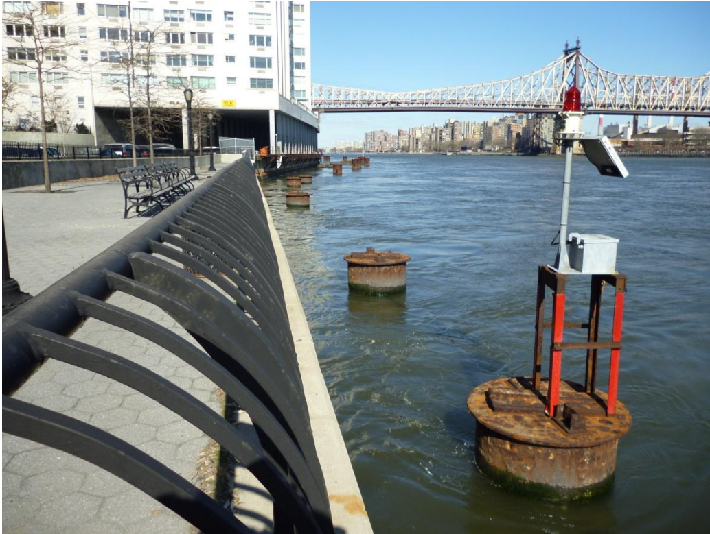
Photo 15 In waterside esplanade opposite East 53 rd Street looking north at ODR drilled shafts/piles left in river that may be reused for EMWE Project.
