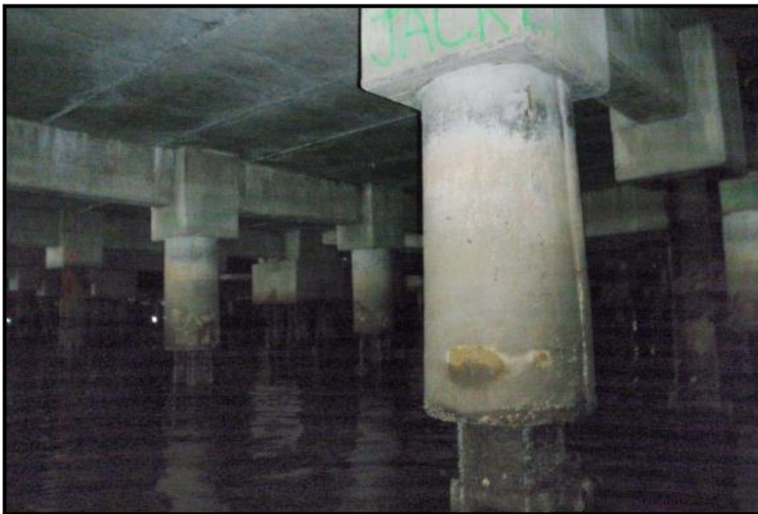
Photo 4: View of the dense pile field under Pier 40. HPA Engineers P.C. 2009
