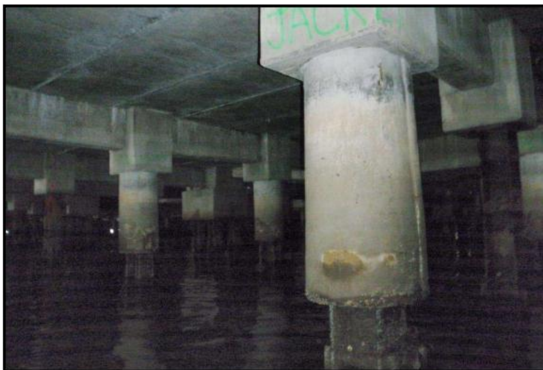
Photo 2. View of the dense pile field under Pier 40. HPA Engineers P.C. 2009
