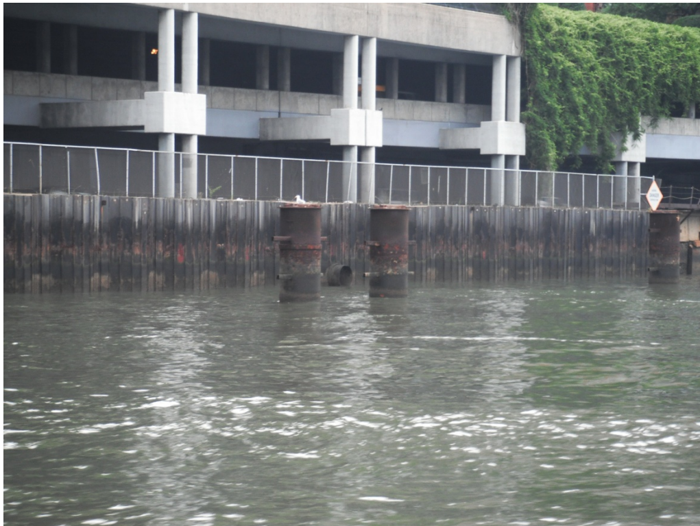
Photo 2 – View of the Sheet Pile Bulkhead. Note outfall between the two caissons.
