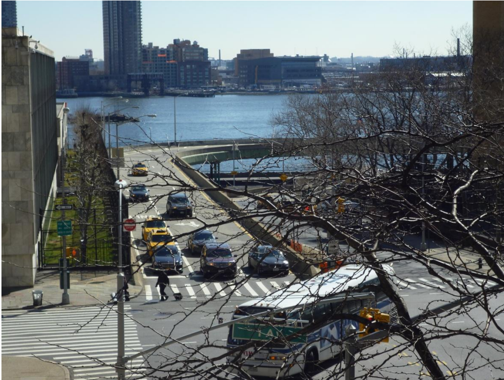
1 2 Photo 5 On Tudor Place looking at East 42 nd Street Ramp. Note elevated curve section of ramp. 3
