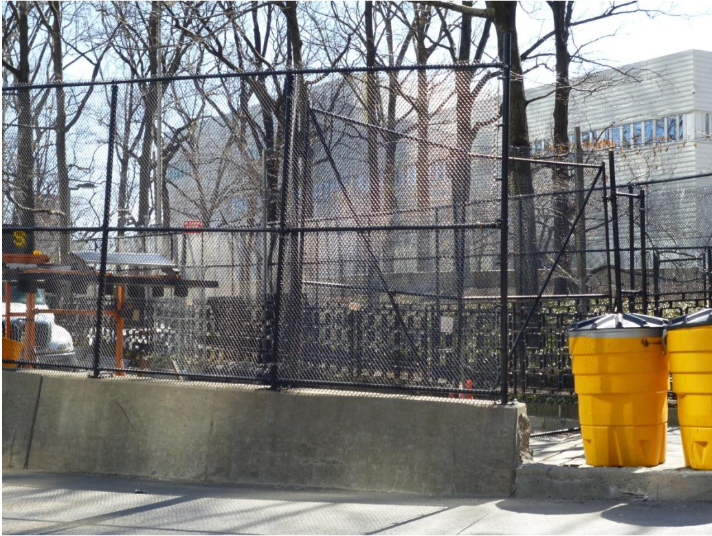
1 2 3 Photo 7 At northwest corner of UN Headquarters property looking southeast at unused section of 4 East 48 th Street ramp between north fence of UN property and extant East 48 th Street ramp.
