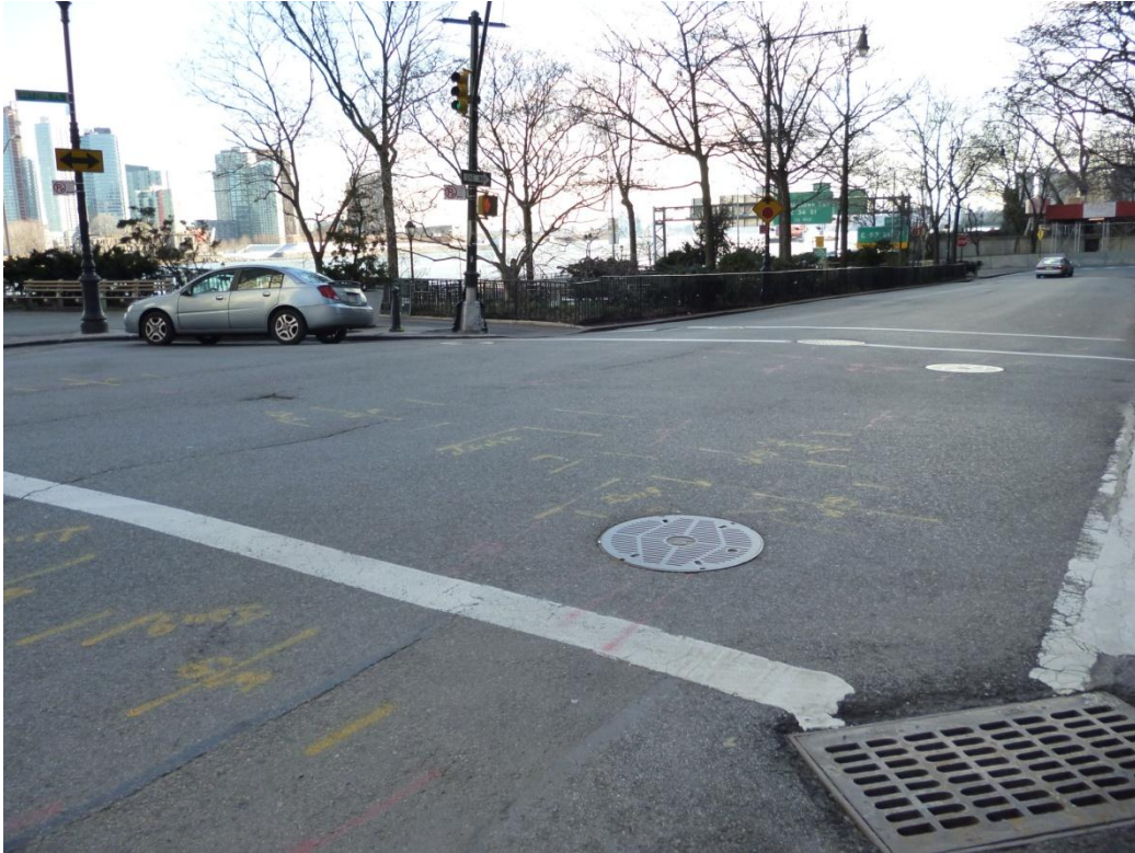
1 2 Photo 19 At terminus of East 54 th Street at Sutton Place looking south-southeast at end of park at 3 East 53 rd Street. Note multiple utility mark-outs on pavement, manholes, and storm drain grate. 4
