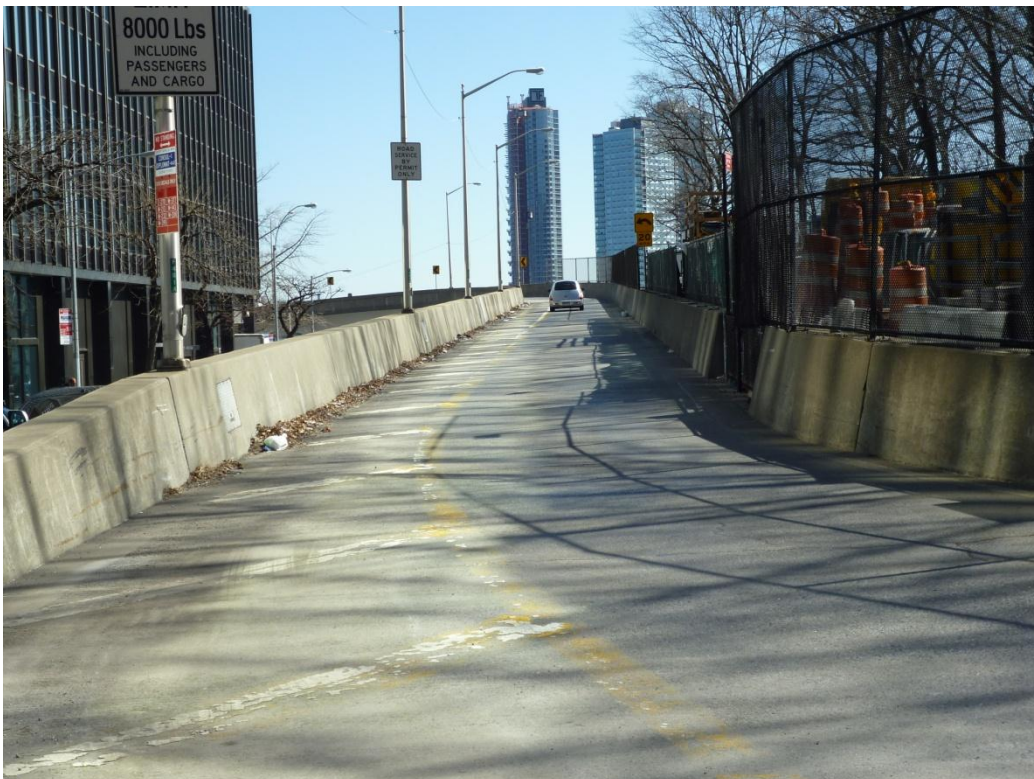
4 5 Photo 6 On first Avenue at northwest corner of UN Headquarters property looking east up East 6 48 th Street FDR Drive northbound entrance ramp.
