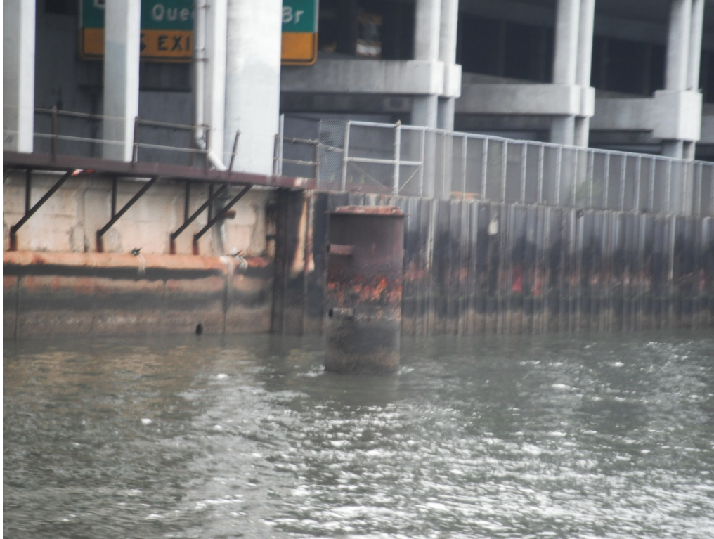
Photo 2 – View of the Sheet Pile Bulkhead. Note outfall between the two caissons.
