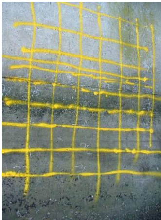
Figure 3-1: Painted grid following a typical cover survey on a concrete element.
