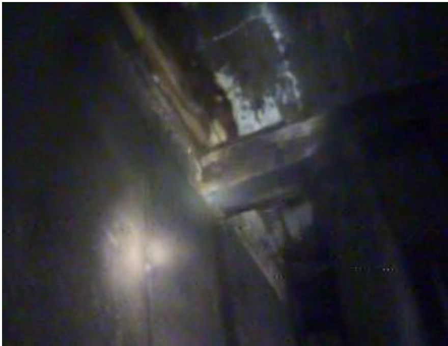
Photo 12- Timber Piles cast into the rearward seawall
