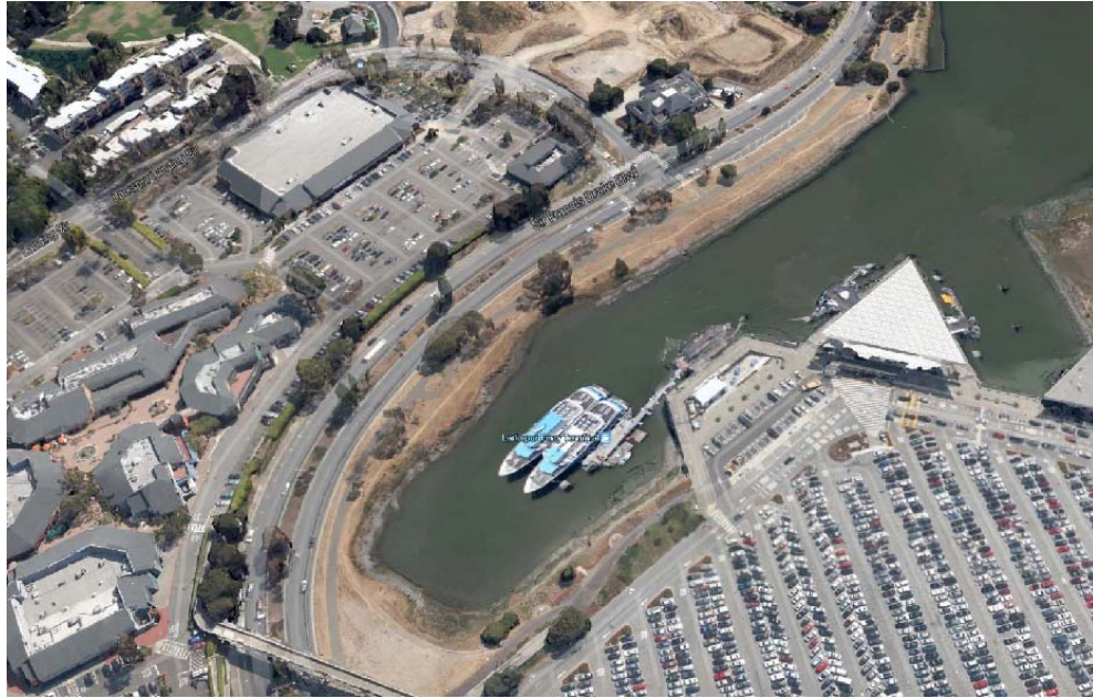
Figure 17. 1: Golden Gate Ferry Larkspur Terminal
